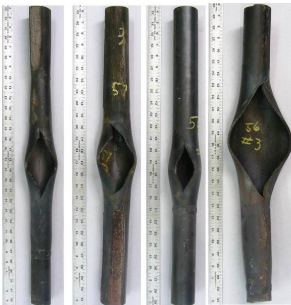
Figure 1. Several secondary tube failures due to short-term overheating during start-up periods
